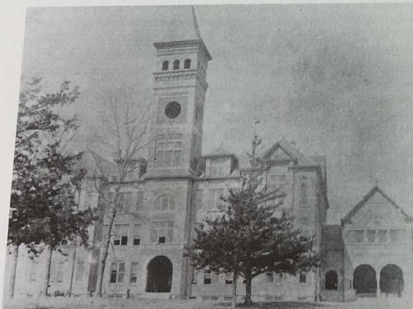
Front elevation in 1894 before fire.
